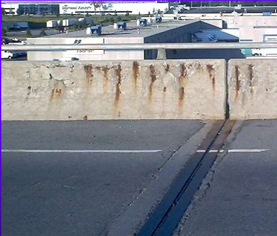
Overall view of the advanced concrete degradation in the barrier wall. Spalling and the remains of uncovered reinforcing steel can be seen.
