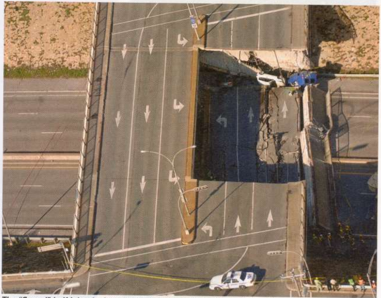
The "flawed" half joint deck structure is no longer used in the UK or Canada
