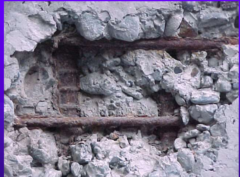
Uniform corrosion
