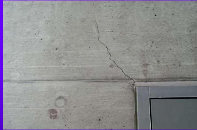
Above the doors
