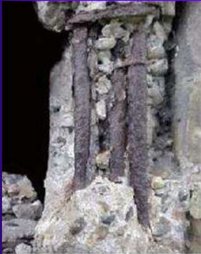
Corrosion of the reinforcing steel in a concrete structure
