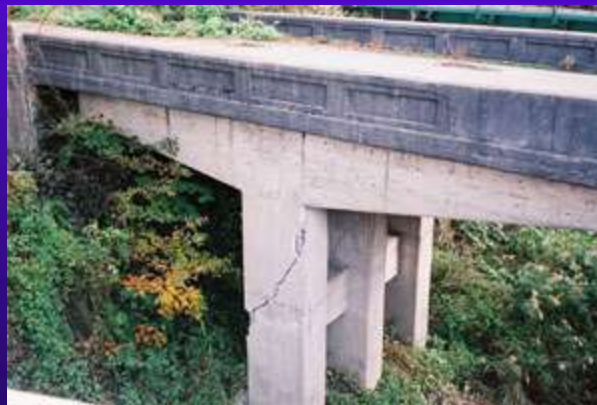
Columns of bridge.
